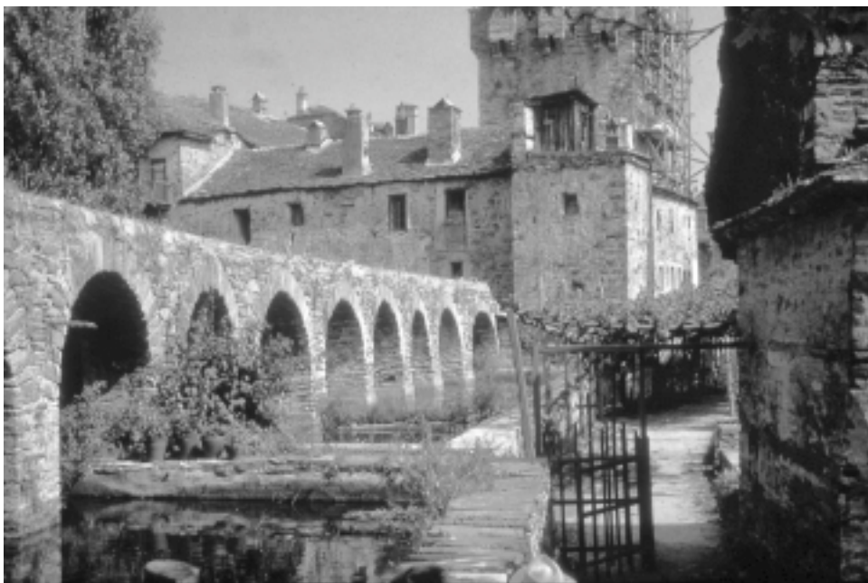
7 Aqueduct at Stavroniketa monastery, Mount Athos (photo: R. Gothóni)
